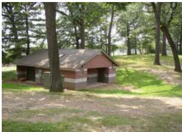
Stadium Park Restrooms
